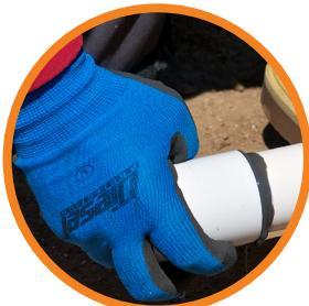
**Work quickly to assemble pipe and fitting immediately after solvent cement is applied and still wet.**
