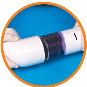
After an even layer of cement is applied, immediately insert pipe into fitting until it bottoms out and hold for approx. 30 seconds. Longer hold time is required in conditions colder than standard ambient temperature. \*
